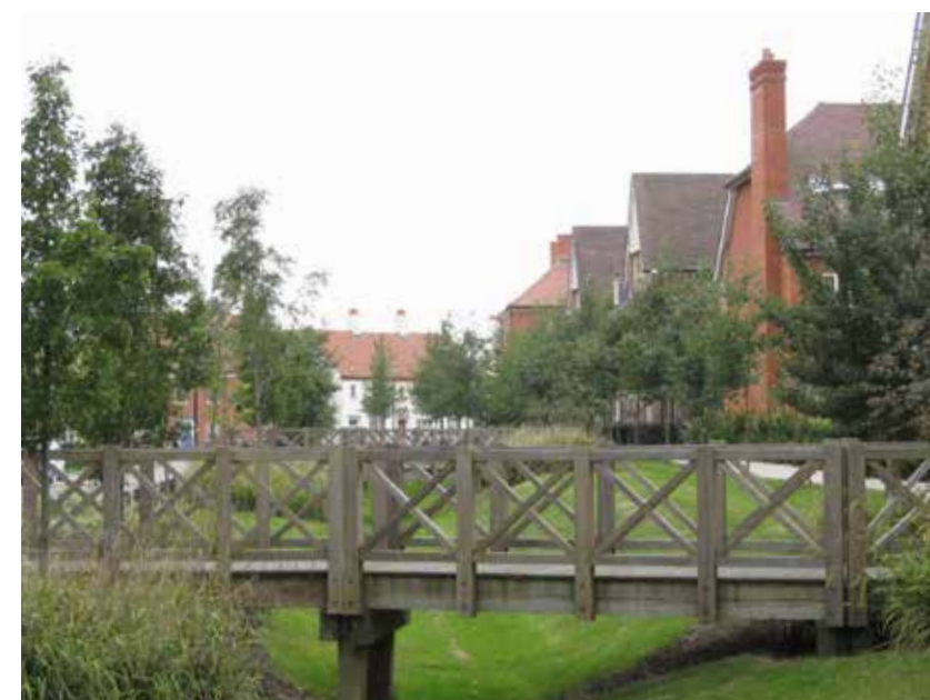
Photo: sustainable drainage channel incorporated into development area
