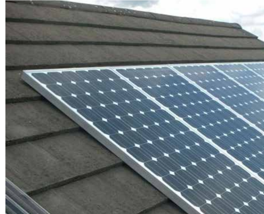
Photo: Photovoltaic roof panels
